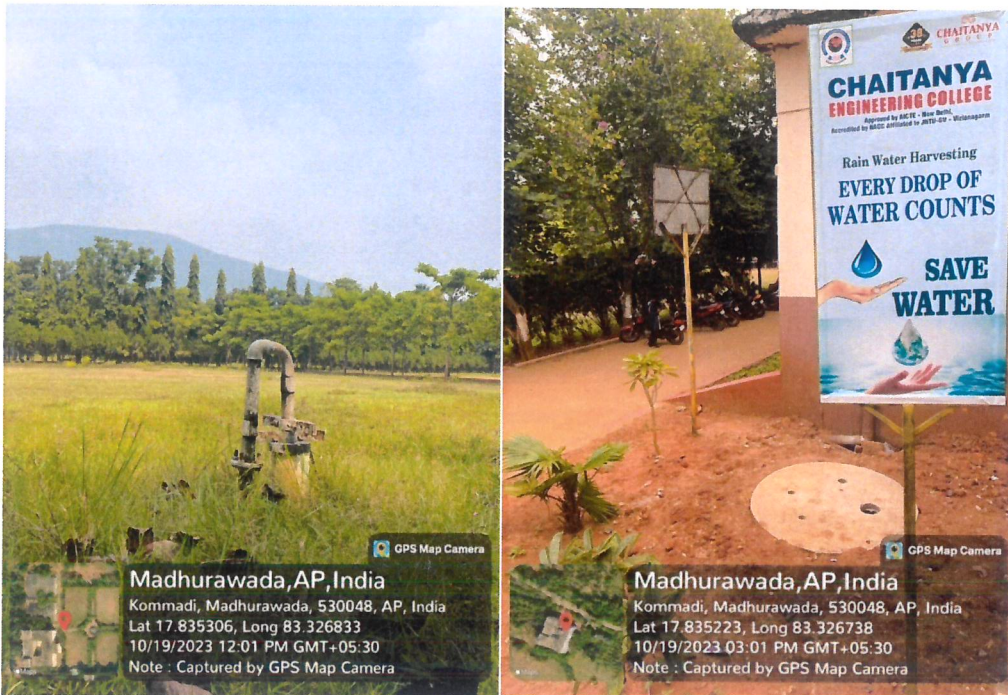
Rain water Harvesting Pit to conserve rain water and Ground water bore well for water resources
